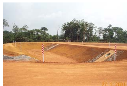
Figure 7.23 Combined temporary and permanent erosion control at Alufer Bel Air, Guinea
