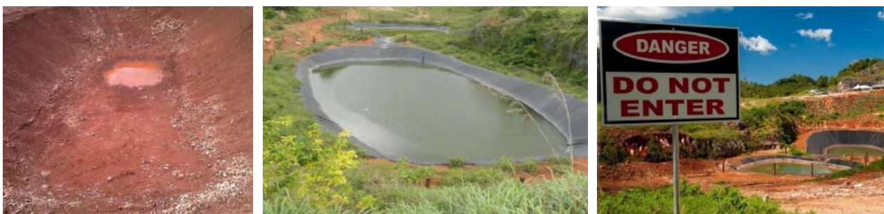
Figure 7.6. Bauxite pit converted to 5 million gallon capacity pond, Tobolski, St Ann, Jamaica
