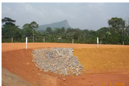
Figure 7.23 Combined temporary and permanent erosion control at Alufer Bel Air, Guinea
