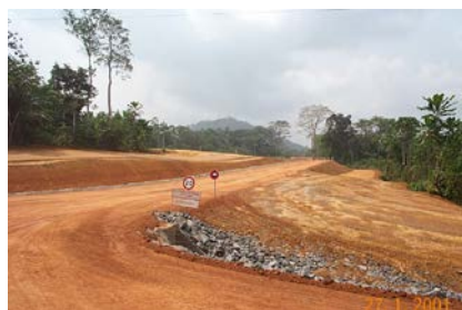
Figure 7.23 Combined temporary and permanent erosion control at Alufer Bel Air, Guinea
